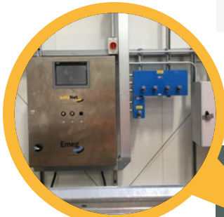
Emeg Remote Operator Logon Panel & Interlocks
